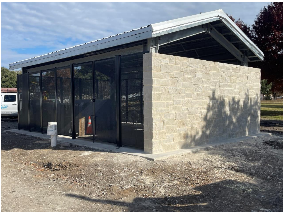
Completed Kidsville Pumphouse
