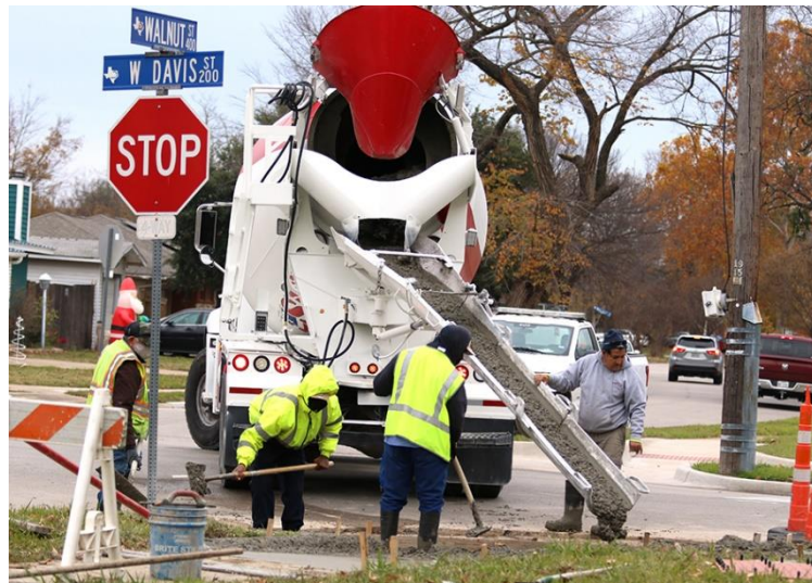
Crews installing ADA ramp on Walnut St.
