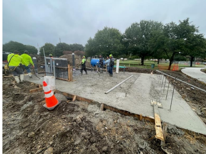
Kidsville Splashpad pump house foundation
