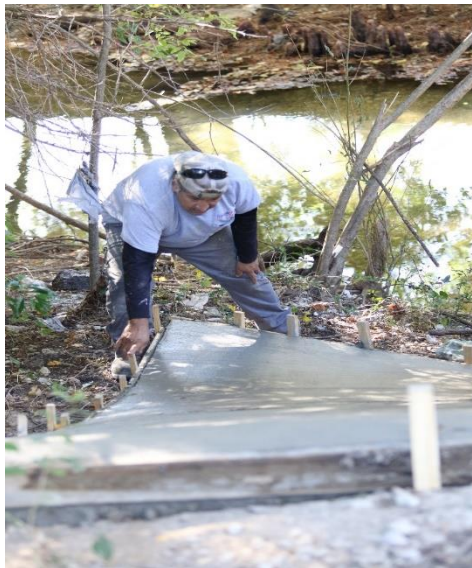
Installing concrete drainage rip rap on Rock Springs Ln.
