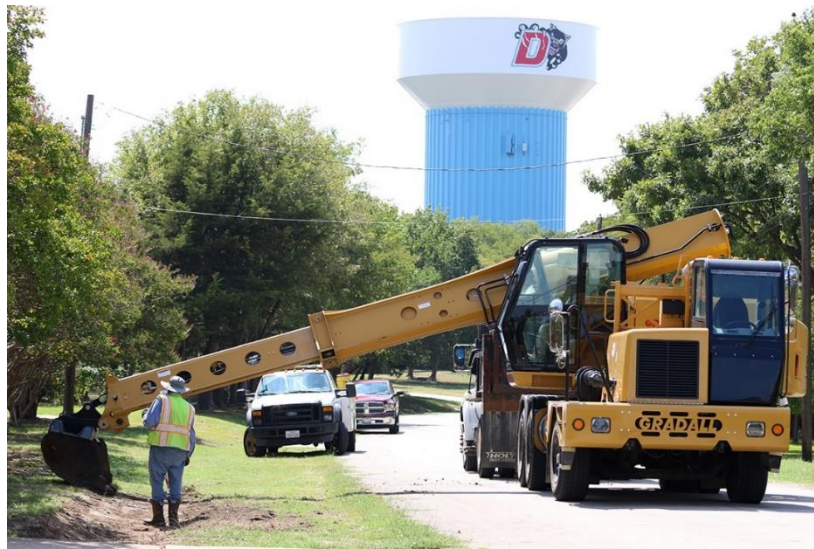
Reshaped open drainage ditch at 106 N. Royal Dr.
