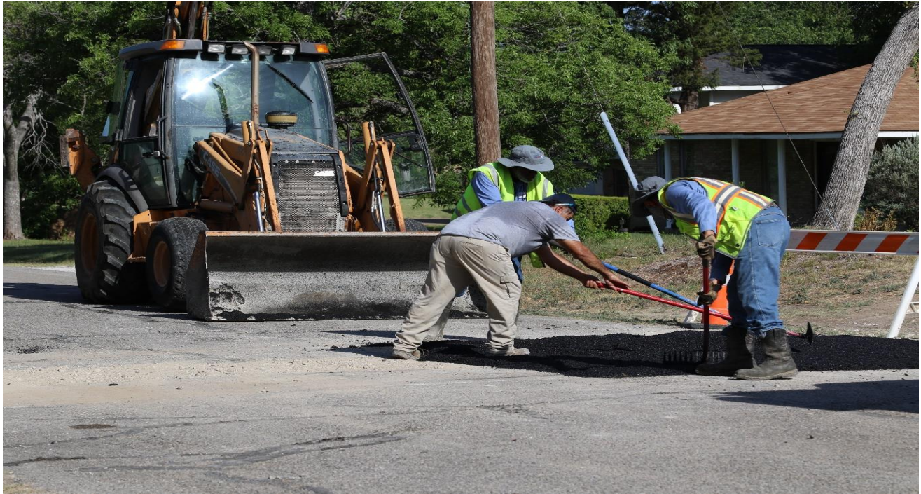
Repairing Utility cut at Rita Lane
