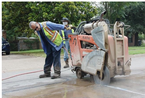
Repairing Utility cut at Kelly Court
