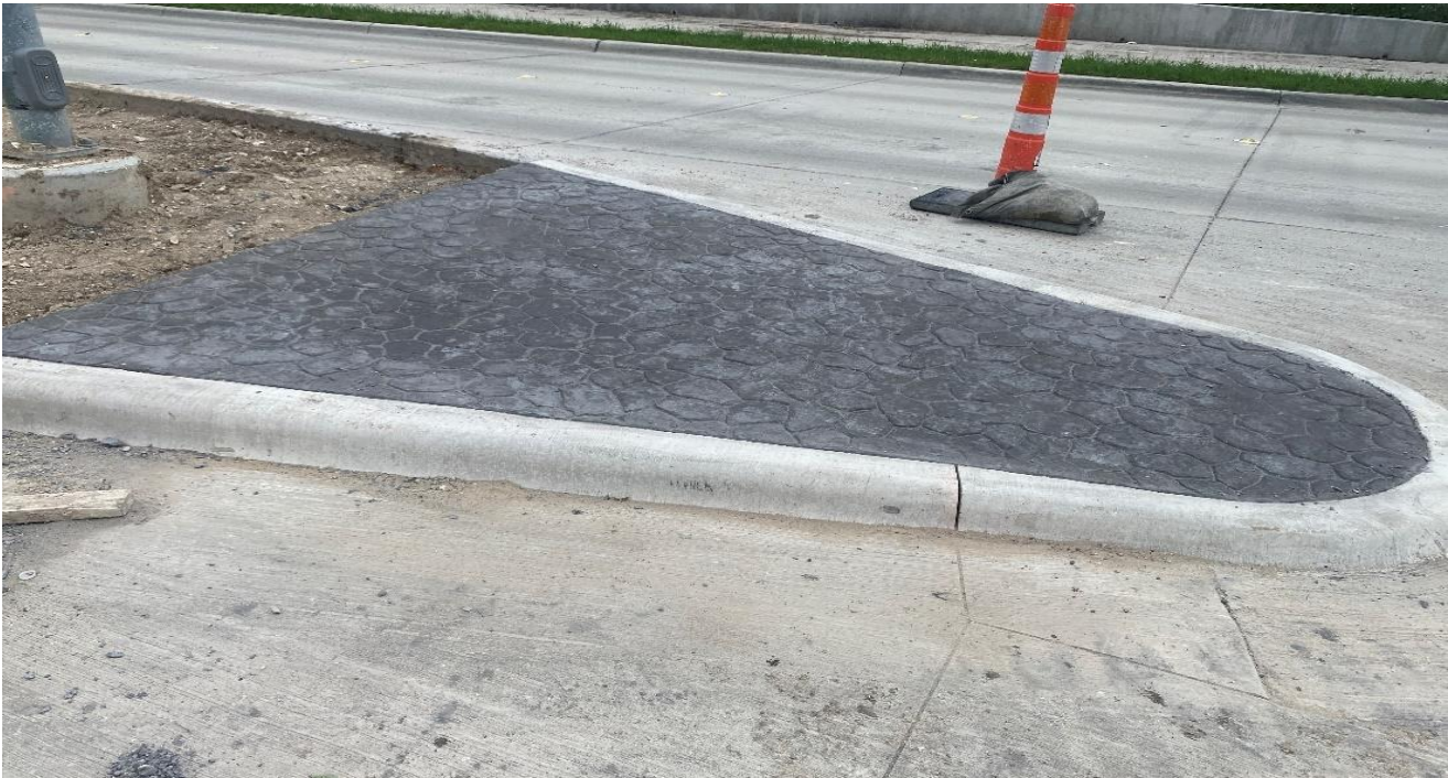
Stamped concrete at median nose
