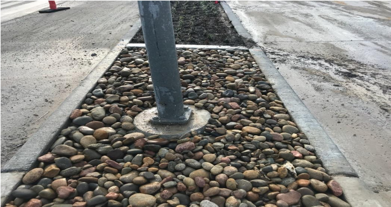
Colorado River rock replacement
