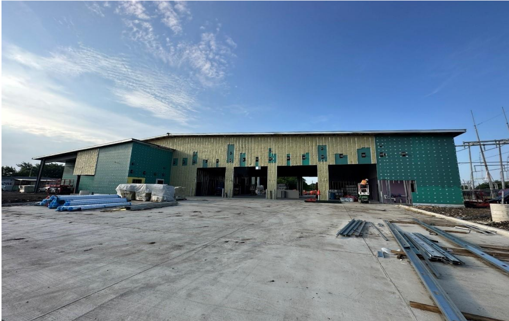
North Elevation Facing Apparatus Bay Entry
