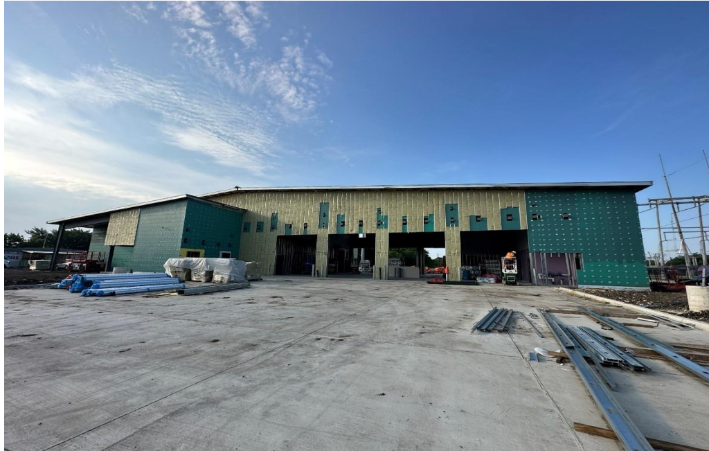
North Elevation Facing Apparatus Bay Entry
