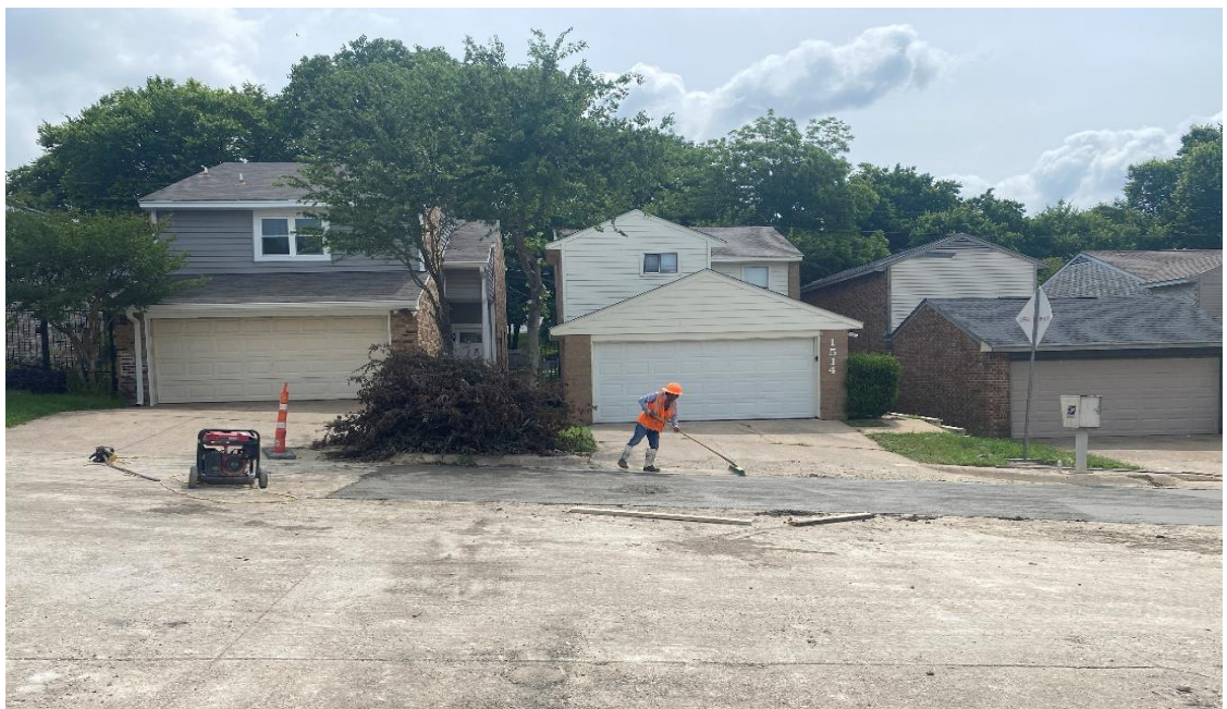
Paving Street Repair Sunset Village Dr.
