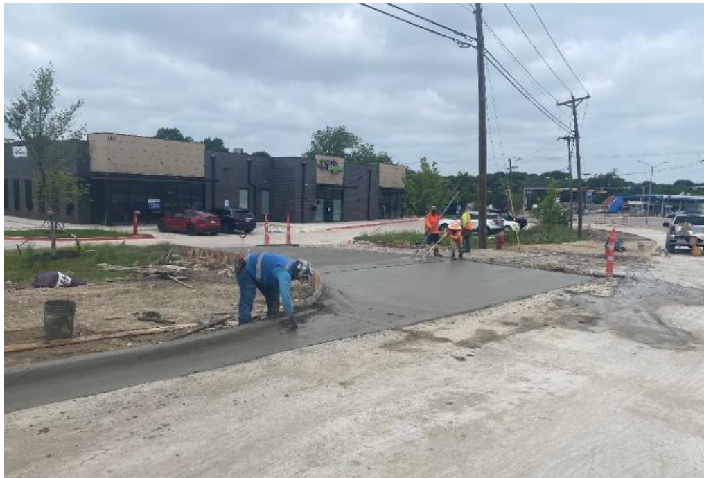
First Half of the Driveway Approach for 102 E. Daniieldale Road
