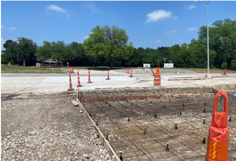
Forms and Rebar for 102 E. Daniieldale Road
