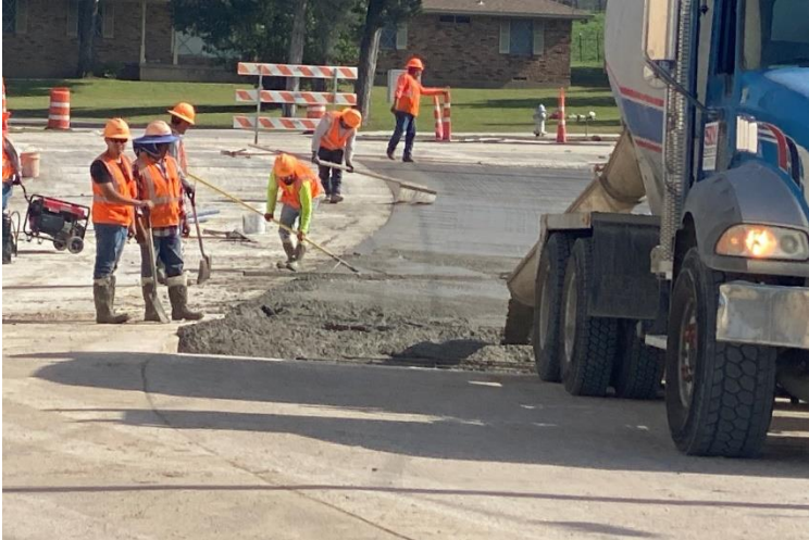
Paving the East Side of Bob Lee Blvd.
