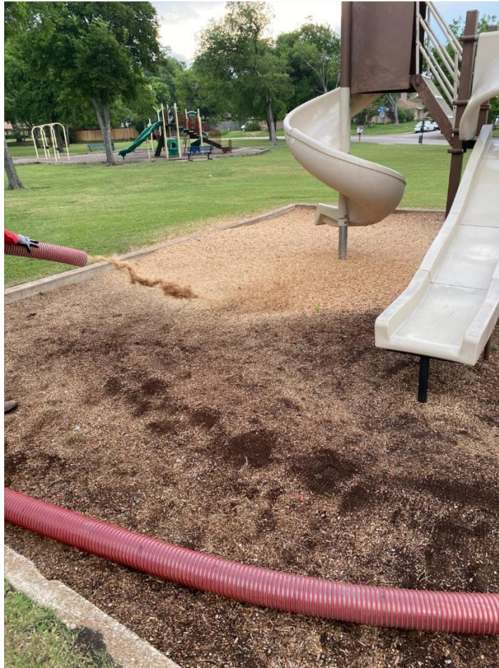
Mulched Safety Surfacing Top-off
