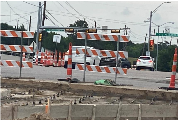
US 67 and E. Daniieldale Road – Connection Ready for Concrete
