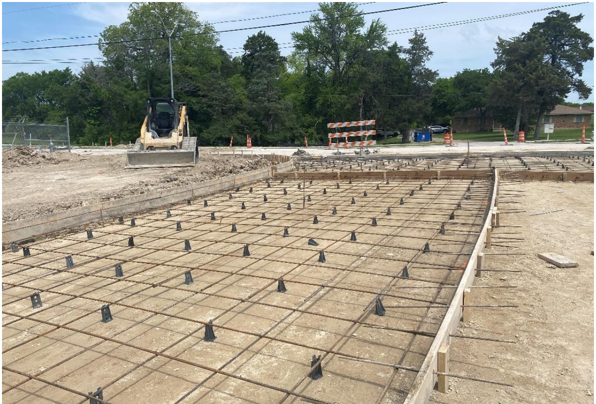
Rebar and Forms – West side of Bob Lee entrance
