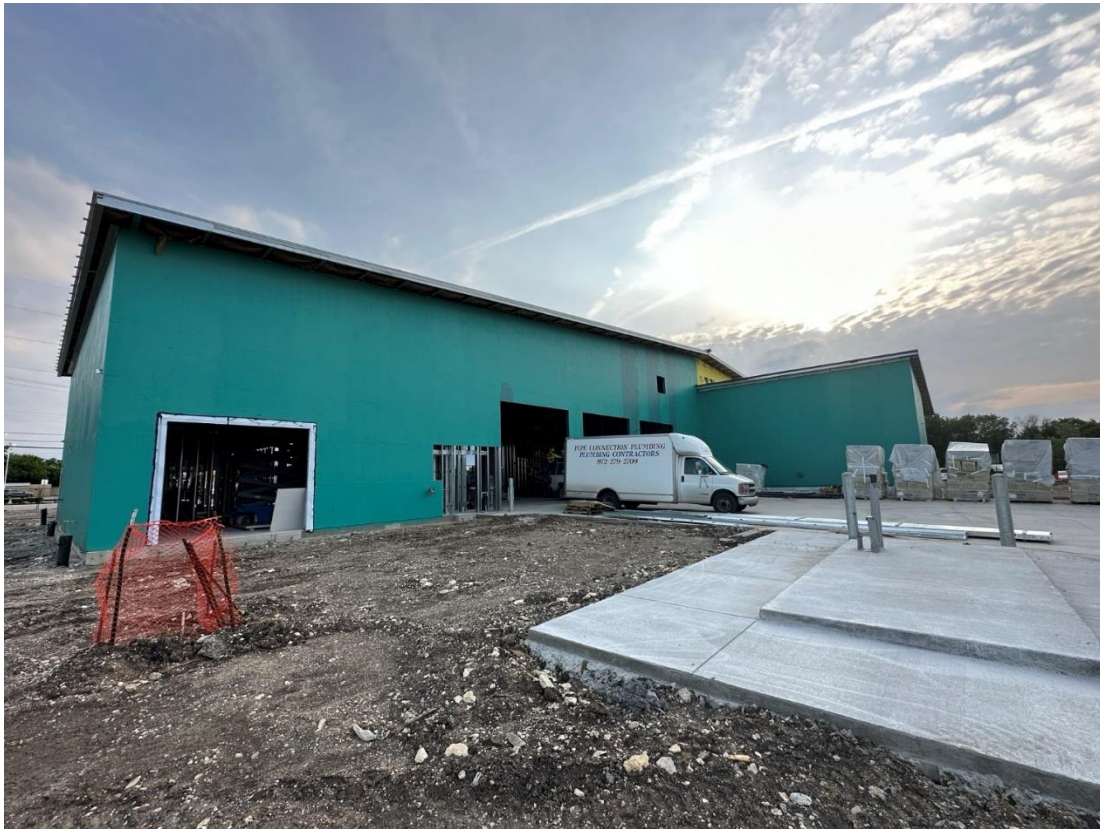
Fire Station 271 – Exterior View
