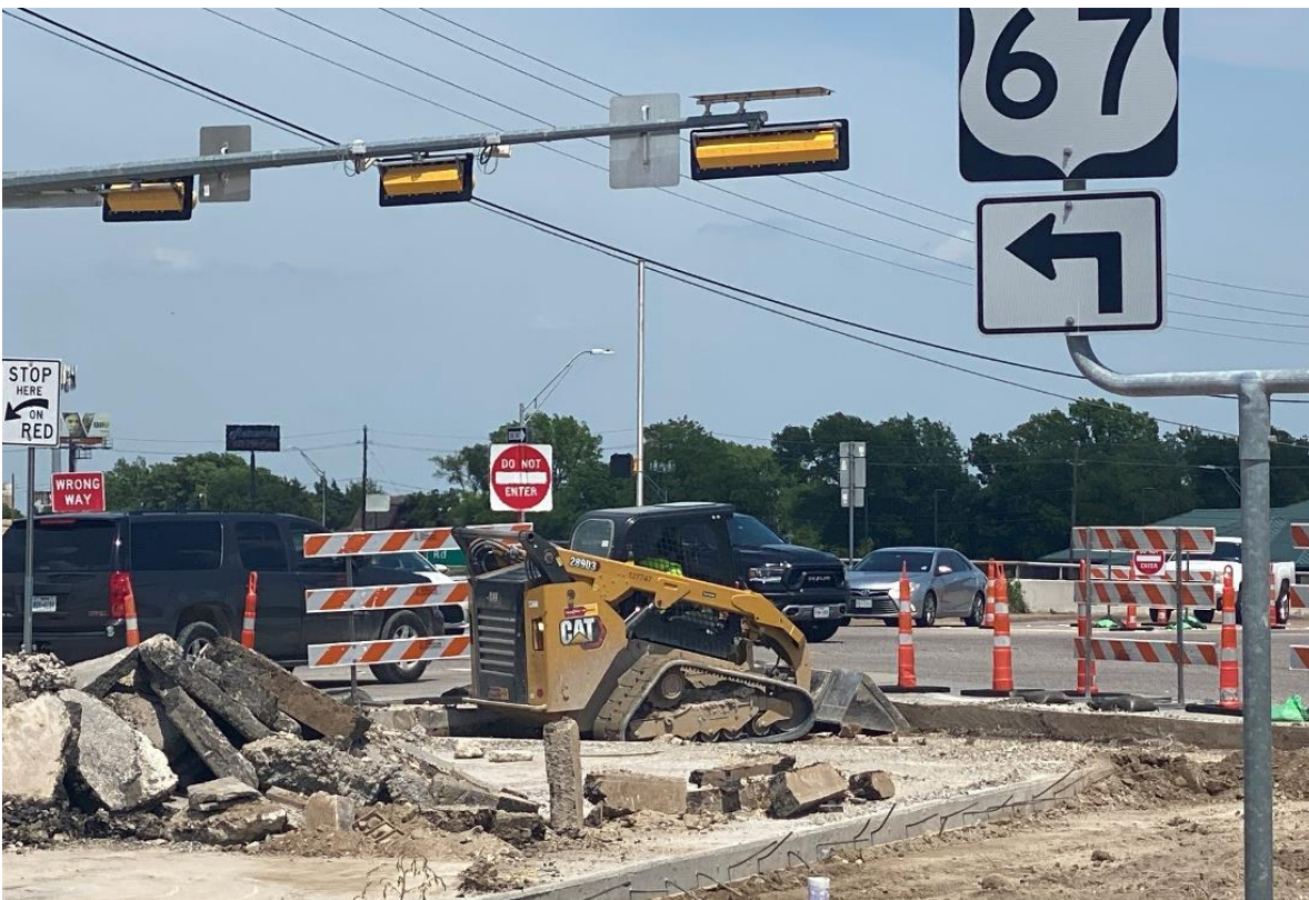
Debris Removal and Grading at U.S. Hwy. 67
