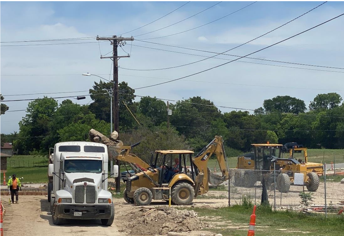
Concrete and Debris Removal from Bob Lee Drop Yard
