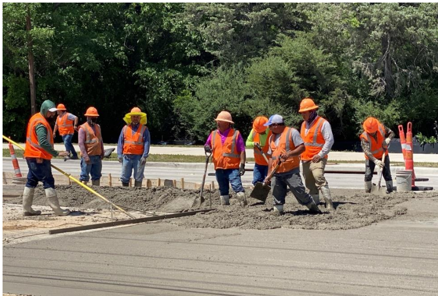
Bob Lee Intersection Paving
