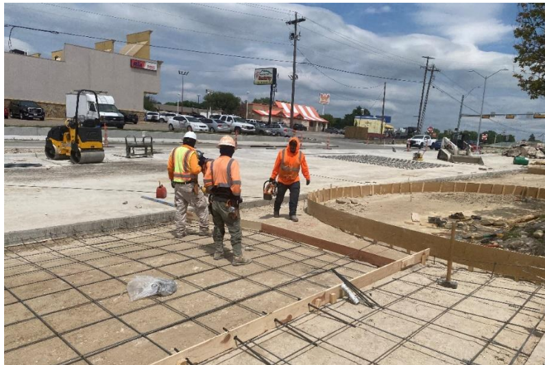
Rebar Placement at 7-11 Driveway
