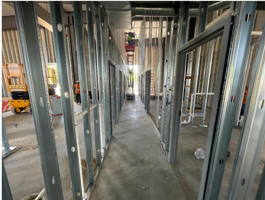
Fire Station 271 – Interior Framing
