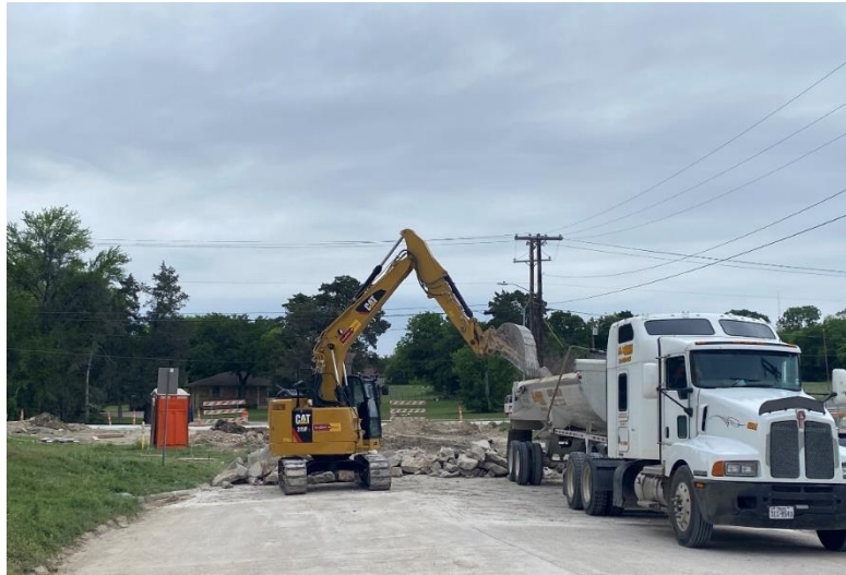
Concrete Removal on Bob Lee
