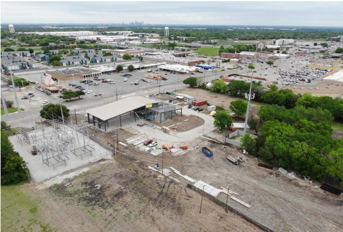
Fire Station 271 – Aerial View of Construction Site
