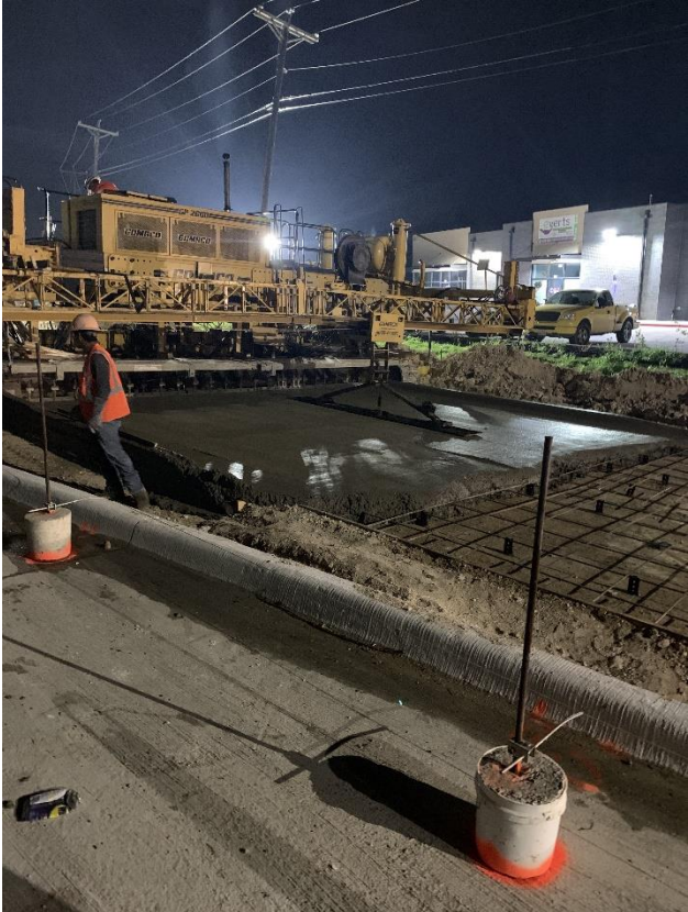
Nighttime Paving Facing Southeast
