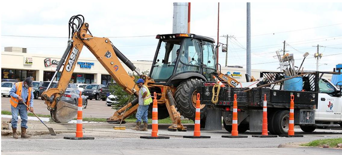
Utility Cut Repair at 332 E. Camp Wisdom
