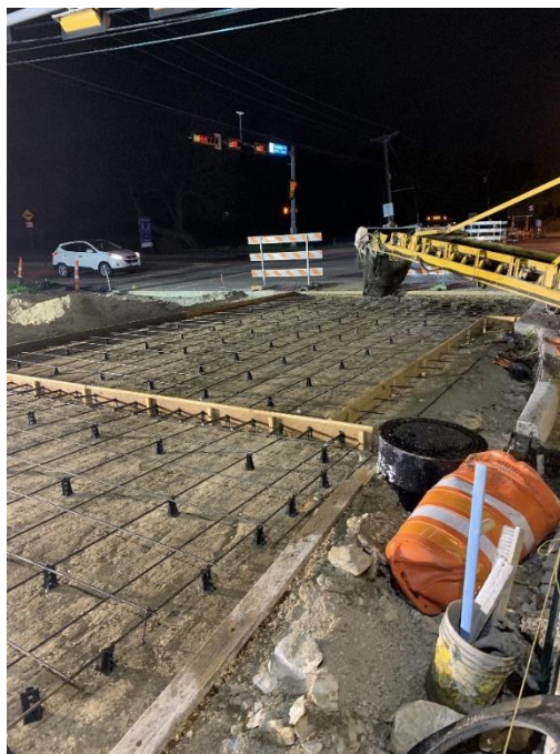
Nighttime Paving of Danieldale Rd Project, Facing Southwest
