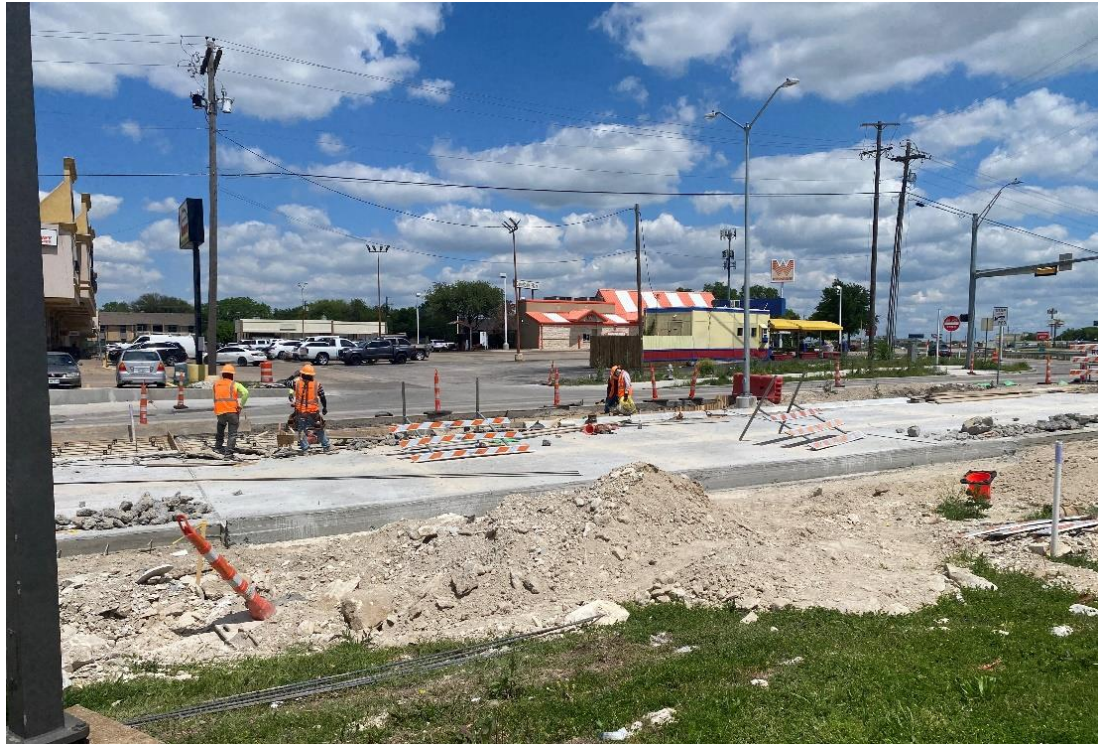
Forming Turn lanes at E. Danieldale and US67 Frontage Rd.
