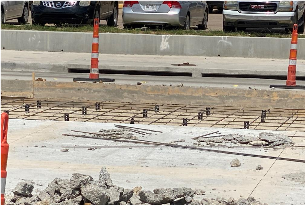
Rebar Placement
