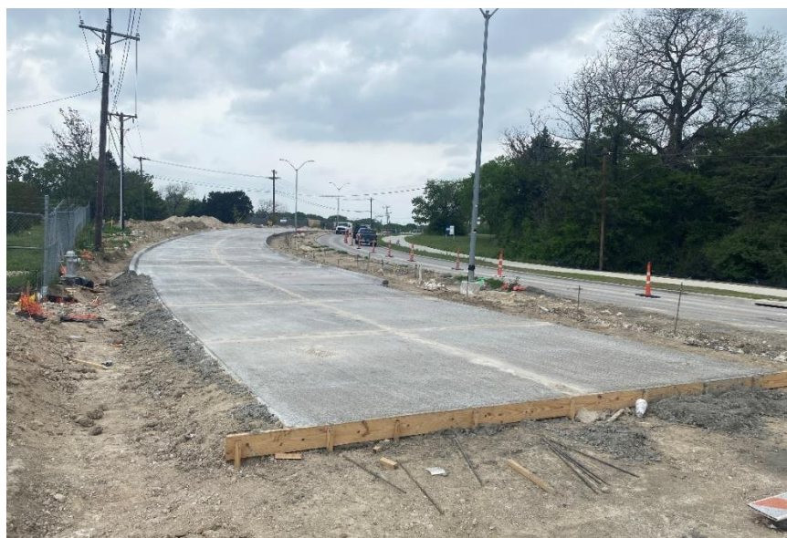
Paving View (Facing West)
