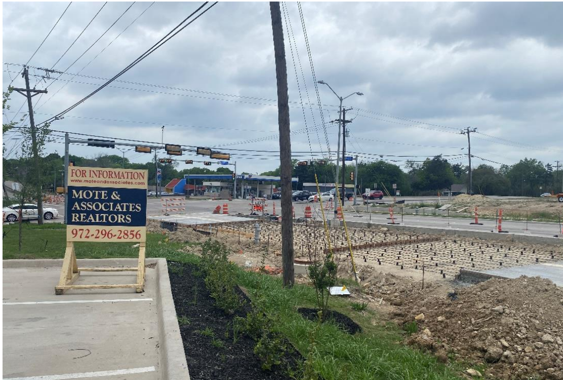
Paving View (Facing Northwest)
