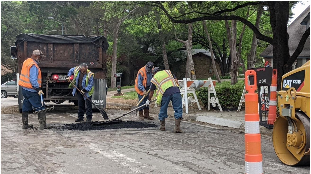
Utility Cut Repair on Swan Ridge
