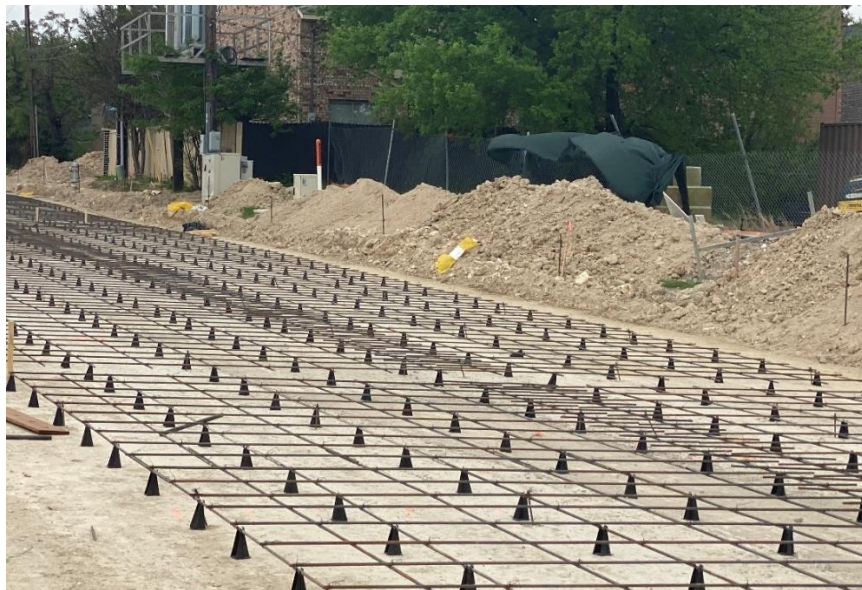
Rebar Placement (Facing East)
