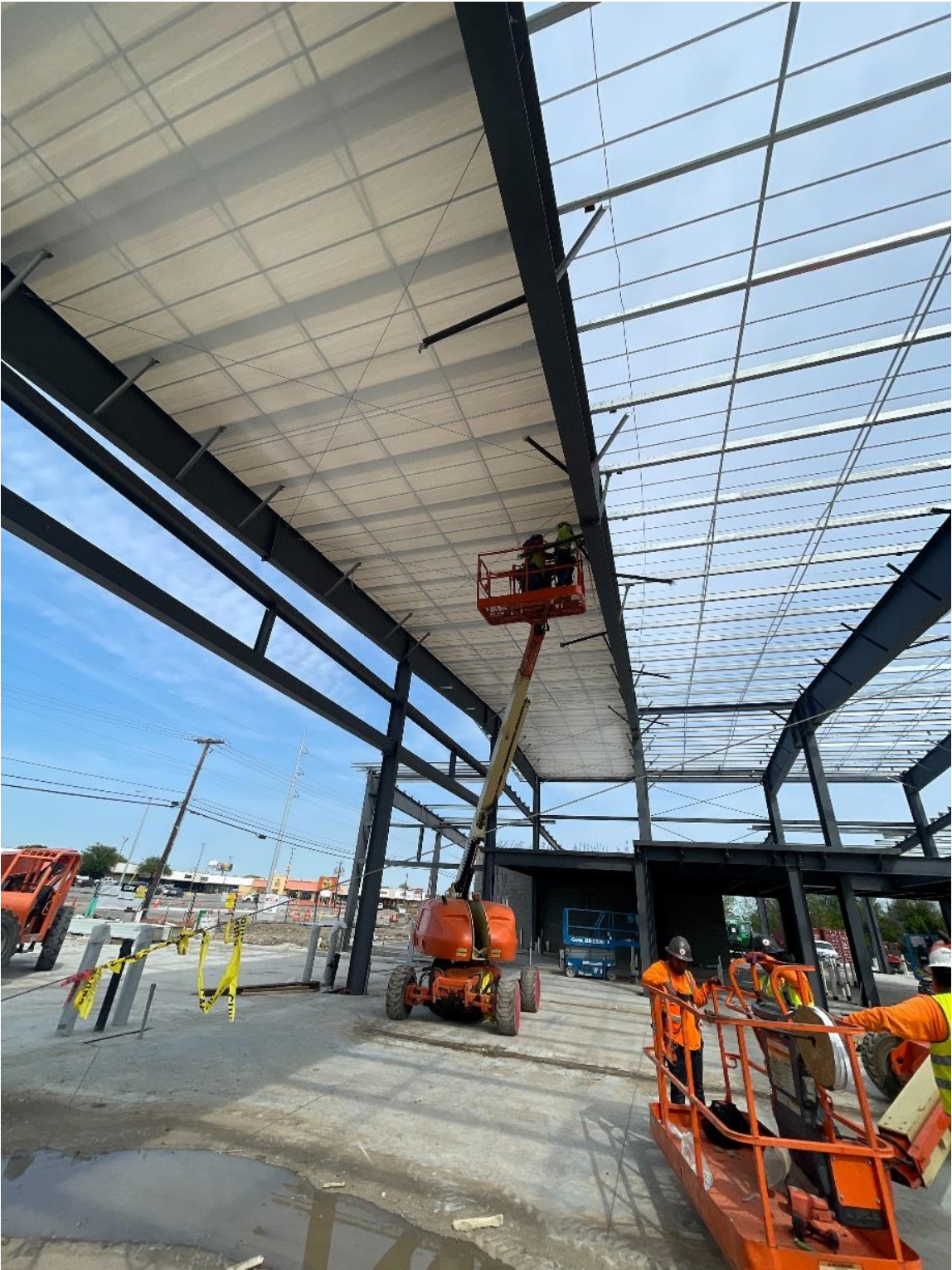
Fire Station 271 Roof Installation
