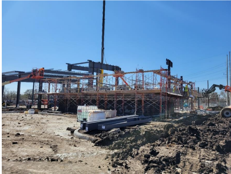
Fire Station 271 building being erected
