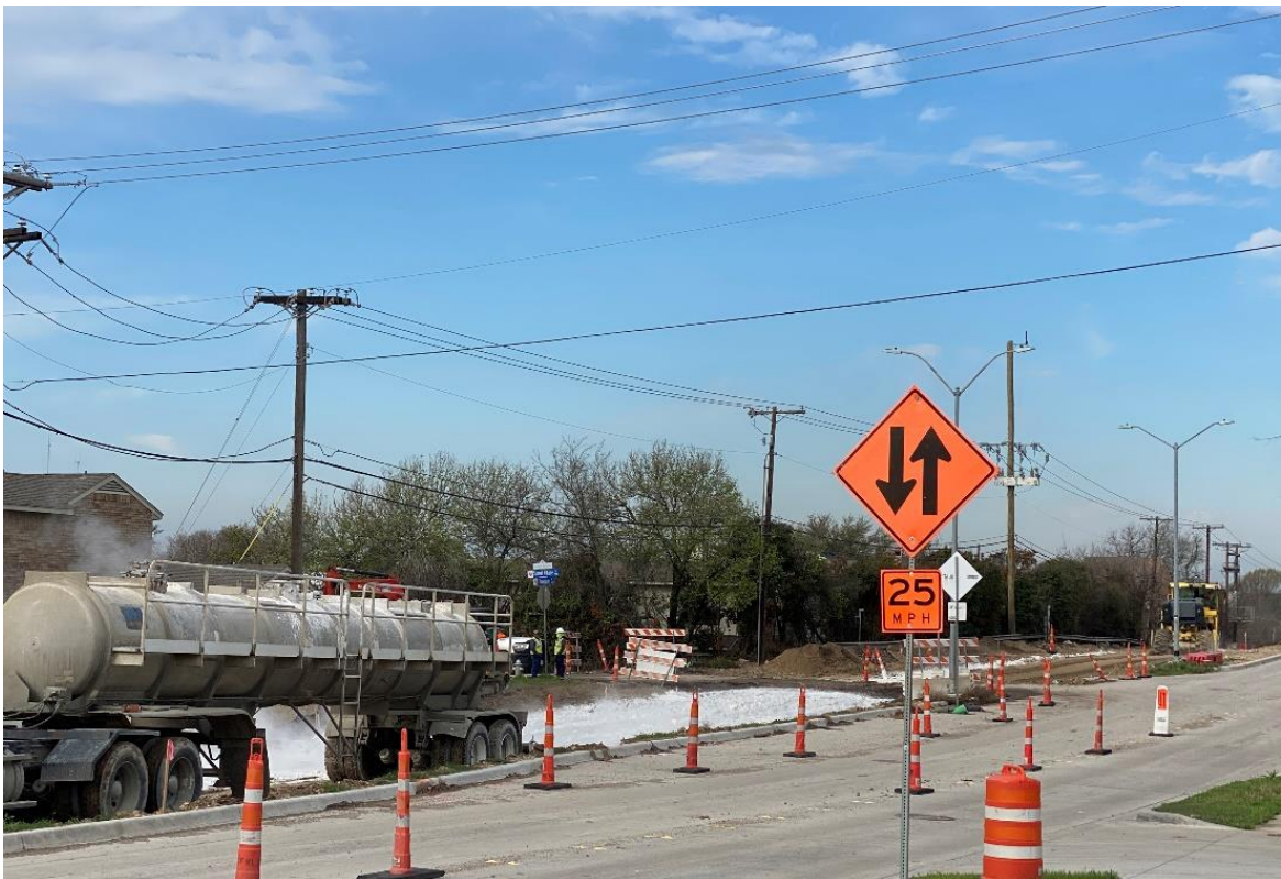
PaveCon Lime Mixing on Danieldale Road
