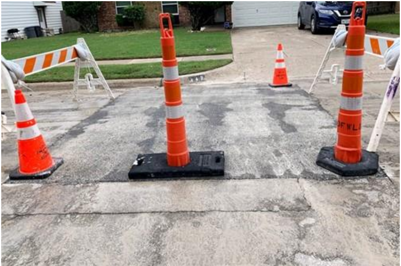
Utility Cut Repair at 442 Kelly
