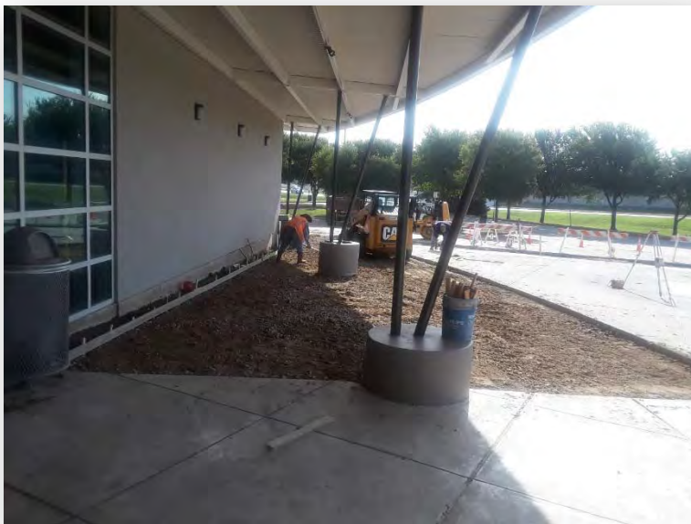
New Patio Construction
