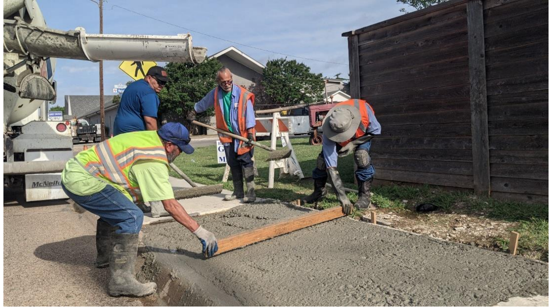
Sidewalk repair at 102 Walnut
