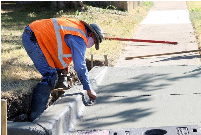
Installing ADA Ramp at 325 Harrington
