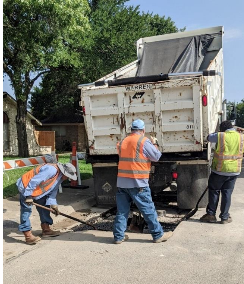
Repairing Utility Cut at 633 Parkwood
