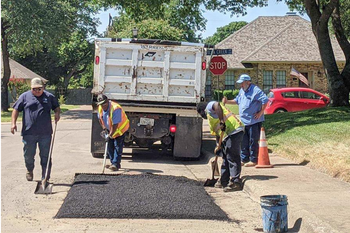
Repairing Asphalt pavement at 603 Villa Creek
