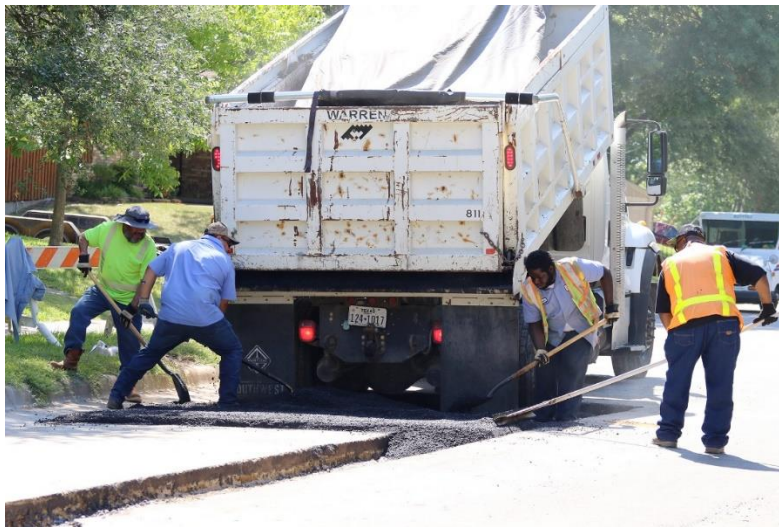
Street repair at 215 Linda Ln.
